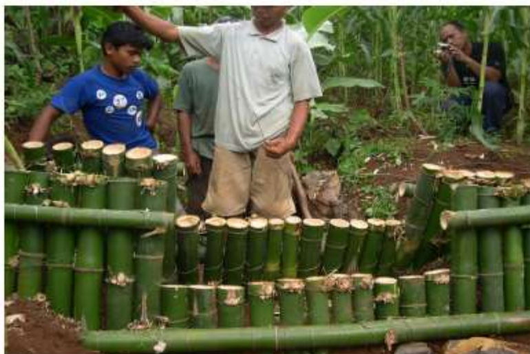
Gambar 4.45. Bio Gully Plug tampak depan di lapangan
