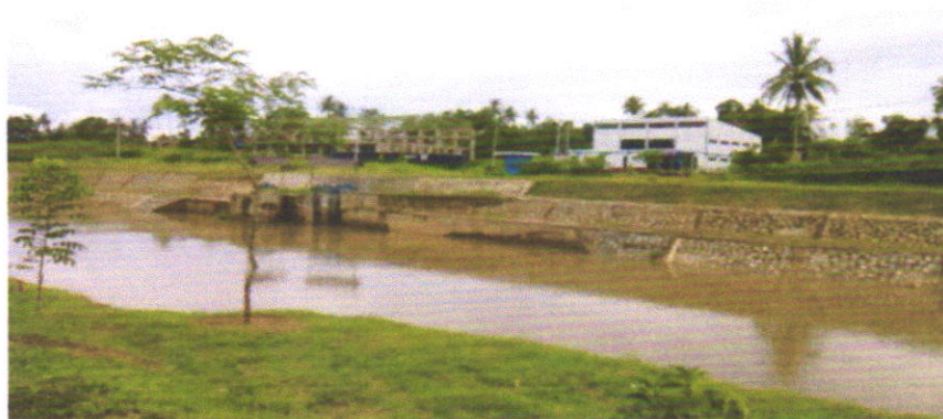
Gambar II-5 Water Treatment Plant (WTP) Kota Payakumbuh
